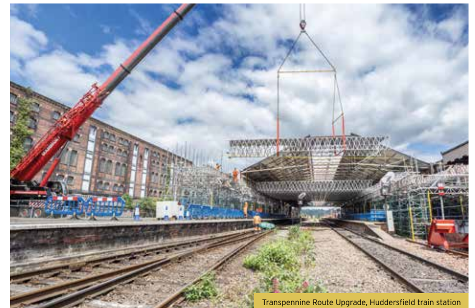
Transpennine Route Upgrade, Huddersfield train station
